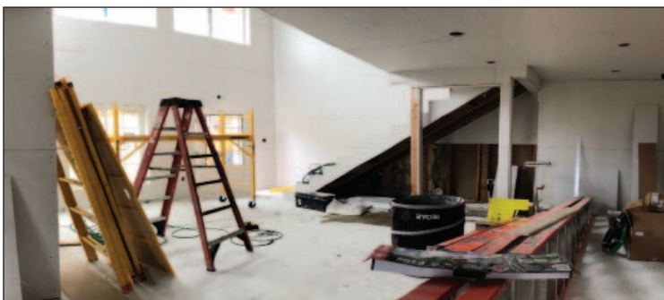
Our multi-purpose family gathering space nears completion.
