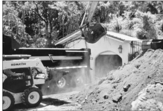
The Mega Construction team excavated, then built a retaining wall in back of the Ronald House (above and right).
