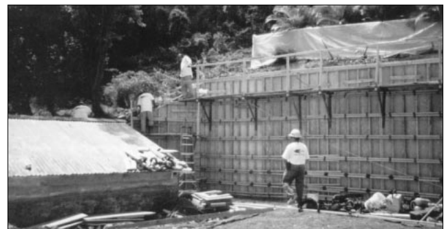
Then the work focused on the front lawn retaining wall (below and left).
